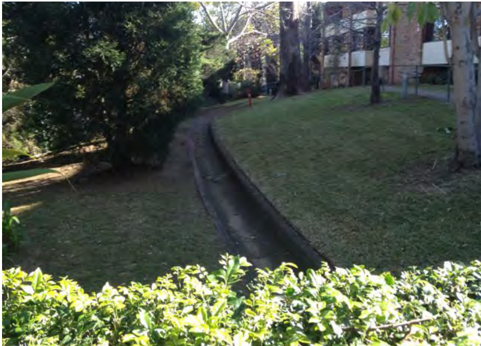
Existing storm water management device on site
