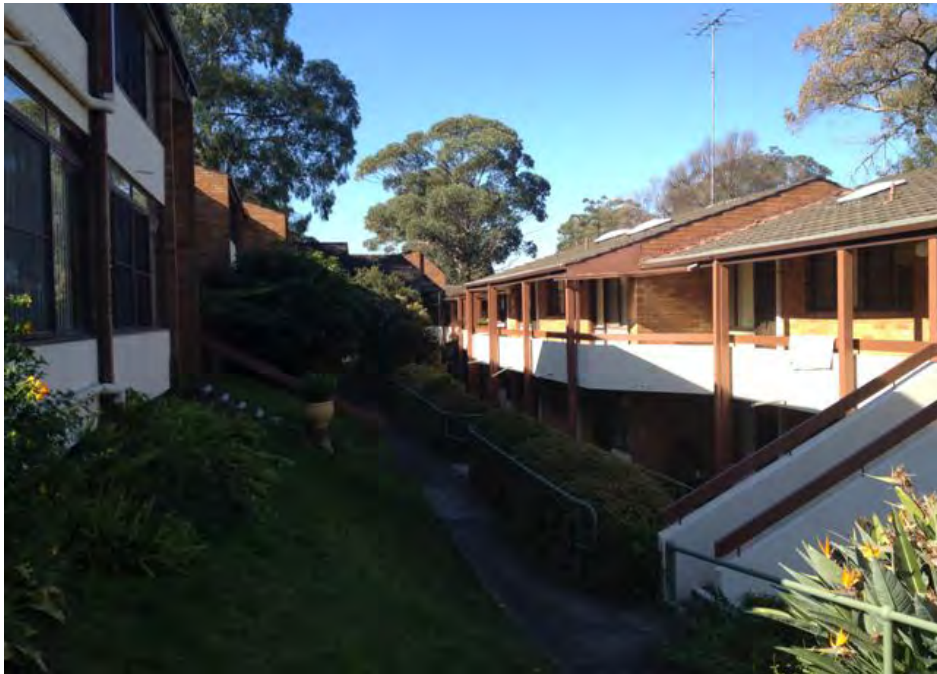
Embankments within site
